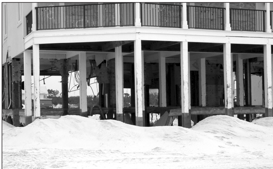
Figure 3. Successful breakaway wall performance
