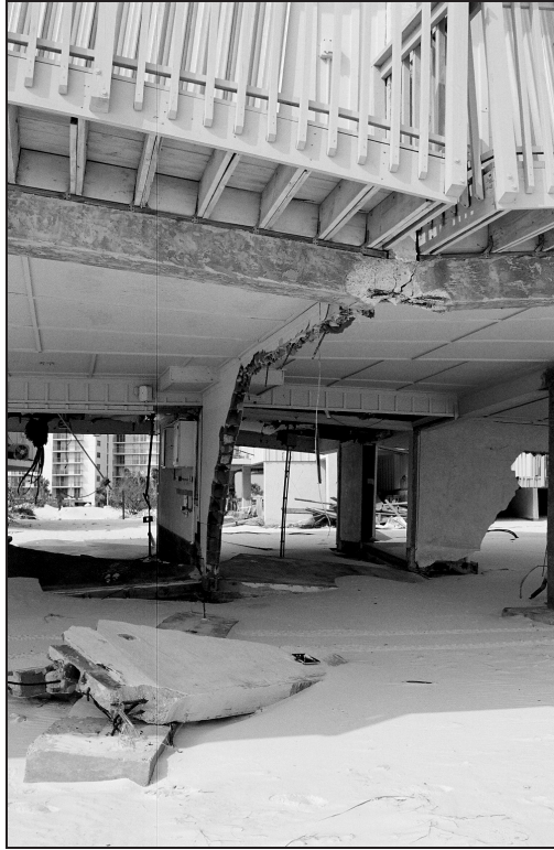
Figure 10. Failure of shore-perpendicular (and shore-parallel) solid foundation walls, and of beam and floor system supported by the shore-perpendicular wall (pre-FIRM structure)
