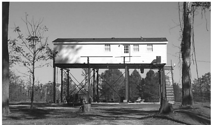
Home elevated on steel pilings.
