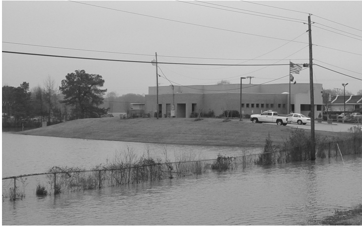
Non-residential building elevated on fill.
