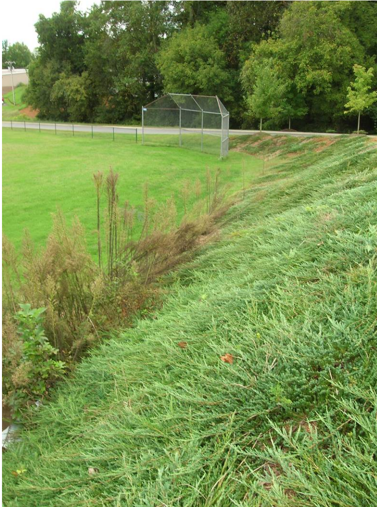
A view of the ditch and the baseball field along which it flows. The ditch flows into a pipe which discharges into UT to Cub Creek (top of photo).
