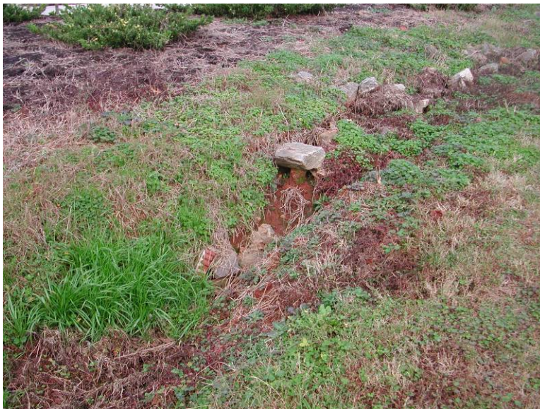
The existing drainage ditch.
