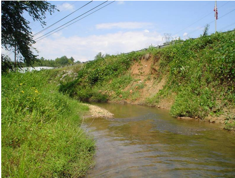
The extreme eroding bank on this outer meander. The guardrail for Foster St. can be seen at the top of the bank.
