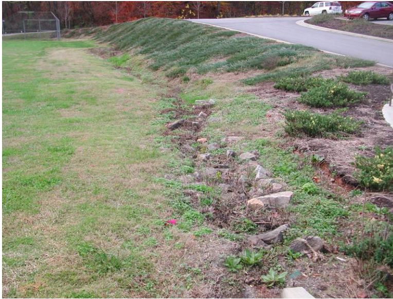
The existing drainage ditch.
