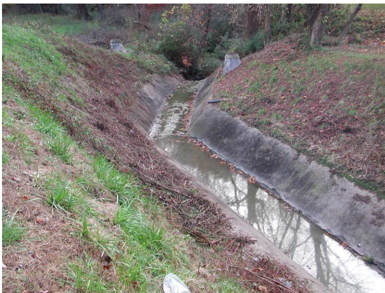
The concrete channel and where it discharges into UT to Cub Creek, looking downstream.
