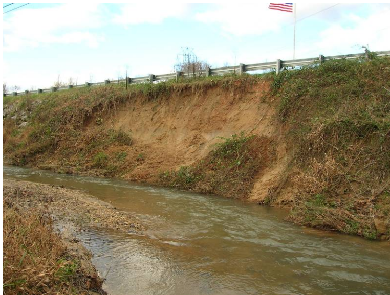
A view of the same bank after the vegetation has died-off, showing the mass wasting occurring on this bank.
