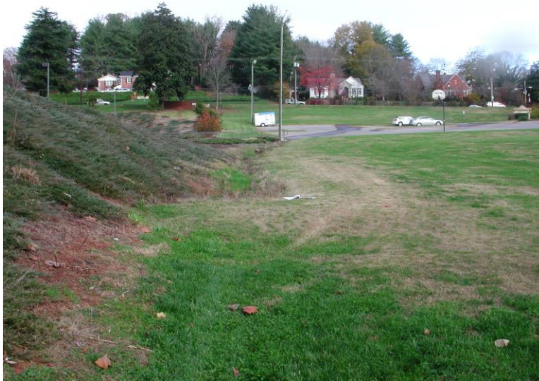
Looking upslope at the ditch and the inlet area.
