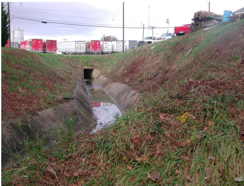
The outfall and concrete channel coming out of the Tyson plant, looking upstream.
