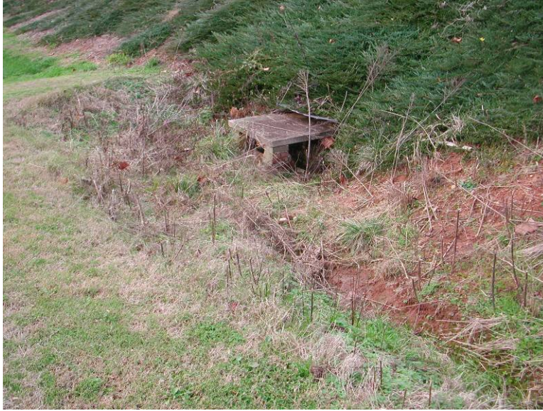
An existing inlet at the base of the ditch could be raised to create a bioretention area.
